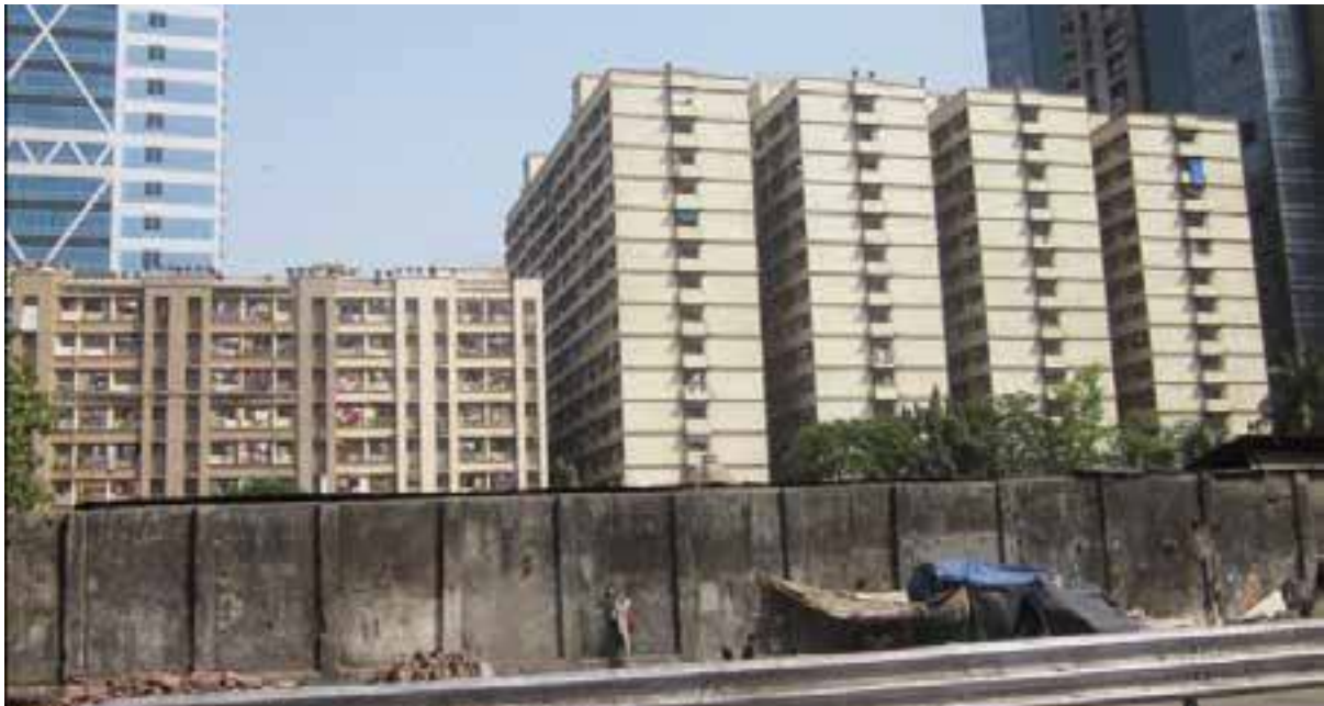
Figure 1.4: Slum redevelopment in Mumbai (blocks of 14 storeys with 3 m distance between them)
